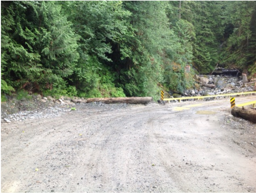
Approach from Right Bank when facing downstream
