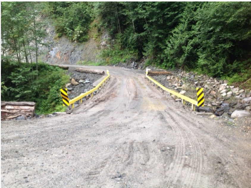
Approach from Left Bank when facing downstream
