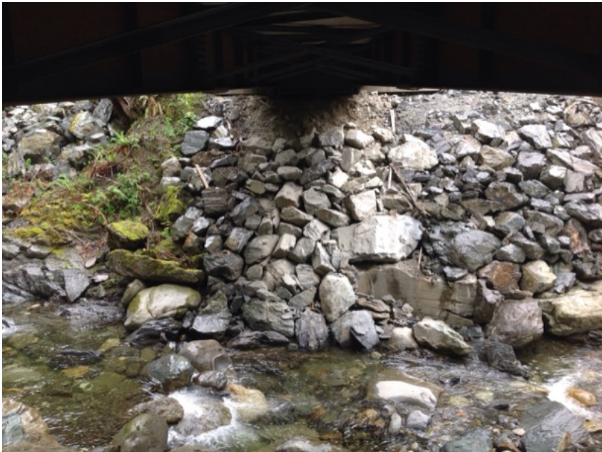
Left Bank Abutment when facing downstream
