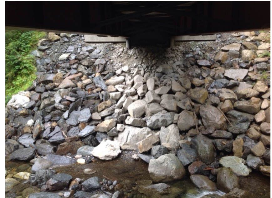
Right Bank Abutment when facing downstream
